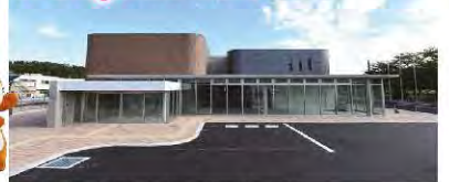
The building facade features specially-made Shigaraki Ware tiles
