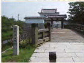
At the time of construction, this rest stop looked like a miniaturized version of Kyoto's Nijo Castle
